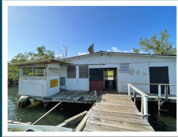
Fishermen's Association La Mela. You can see the raised roof and the “escamadero” about to collapse.
